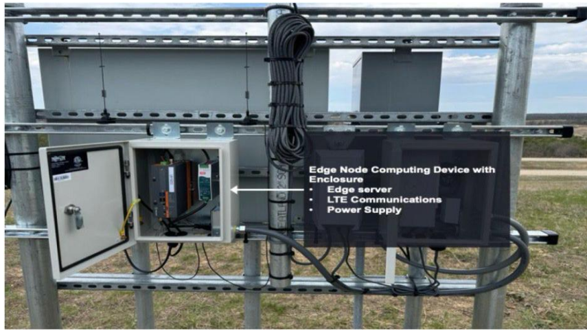
Ground Radar Tower Base Displaying the Power Supply and Serer Location
